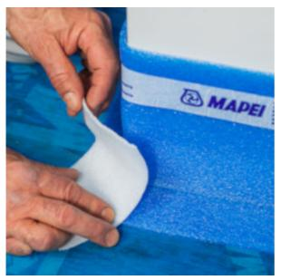
Cut and apply Mapesilent Tape in all the corners and along the overlaps of **Mapesilent Band R** and **Mapesilent** Roll around the blended-in areas of Mapesilent Band R to guarantee that the joints are perfectly protected
