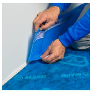
Apply **Mapesilent Band R** around the perimeter of the room, removing the protective film on the reverse side
