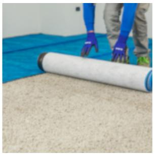
Unroll the sheets of **Mapesilent Roll**, place it against the bottom of the wall and start laying it with the fibre side (the light-coloured side) underneath, following the longer side of the room. Lay the successive rolls by overlapping the side border (approximately 5 cm), to guarantee the continuity of the fiber side
