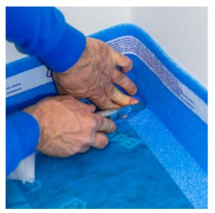
At the corners, cut the lower horizontal part of  ${\it Mape silent}$   ${\it Band}$   ${\it R}$  where necessary
