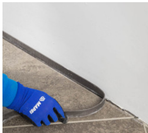
Spread the adhesive on Mapesonic CR and bond the new floor finish
