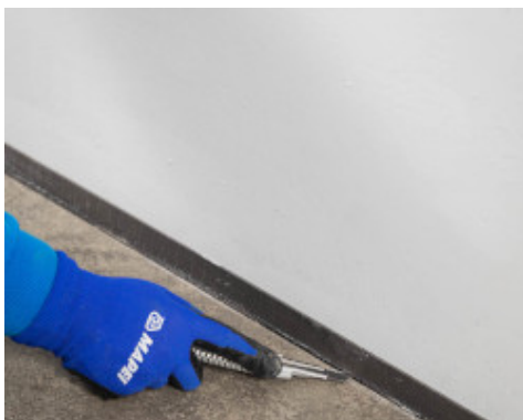
Once the grout has hardened, trim the perimeter of the Mapesonic Strip to remove the excess
