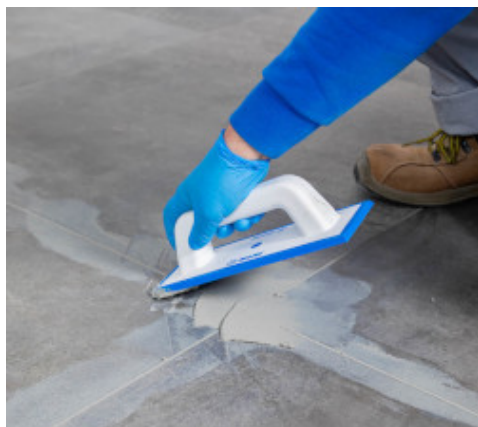
Grout the surface of the room
