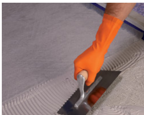
Applying a first layer of Monolastic welded with Mapetex Sel N on a new screed
