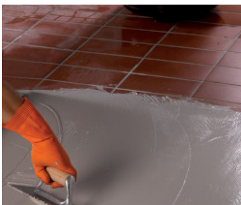
Applying a second layer of Monolastic on Mapenet 150
